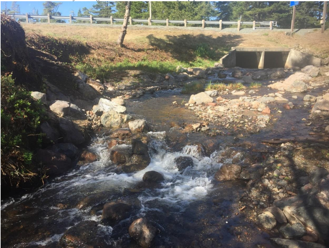
Photo 33- SC#E3 – Modified roughened chute below culvert jump pool. 10-11-2017
