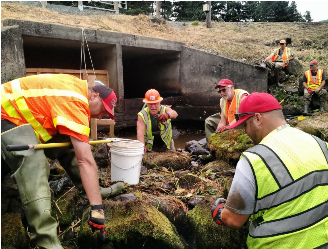
Photo 29- SC #E3 – ODOT modifying baffles for lamprey passage. Water diversion pipe on left. 8-11-2017
