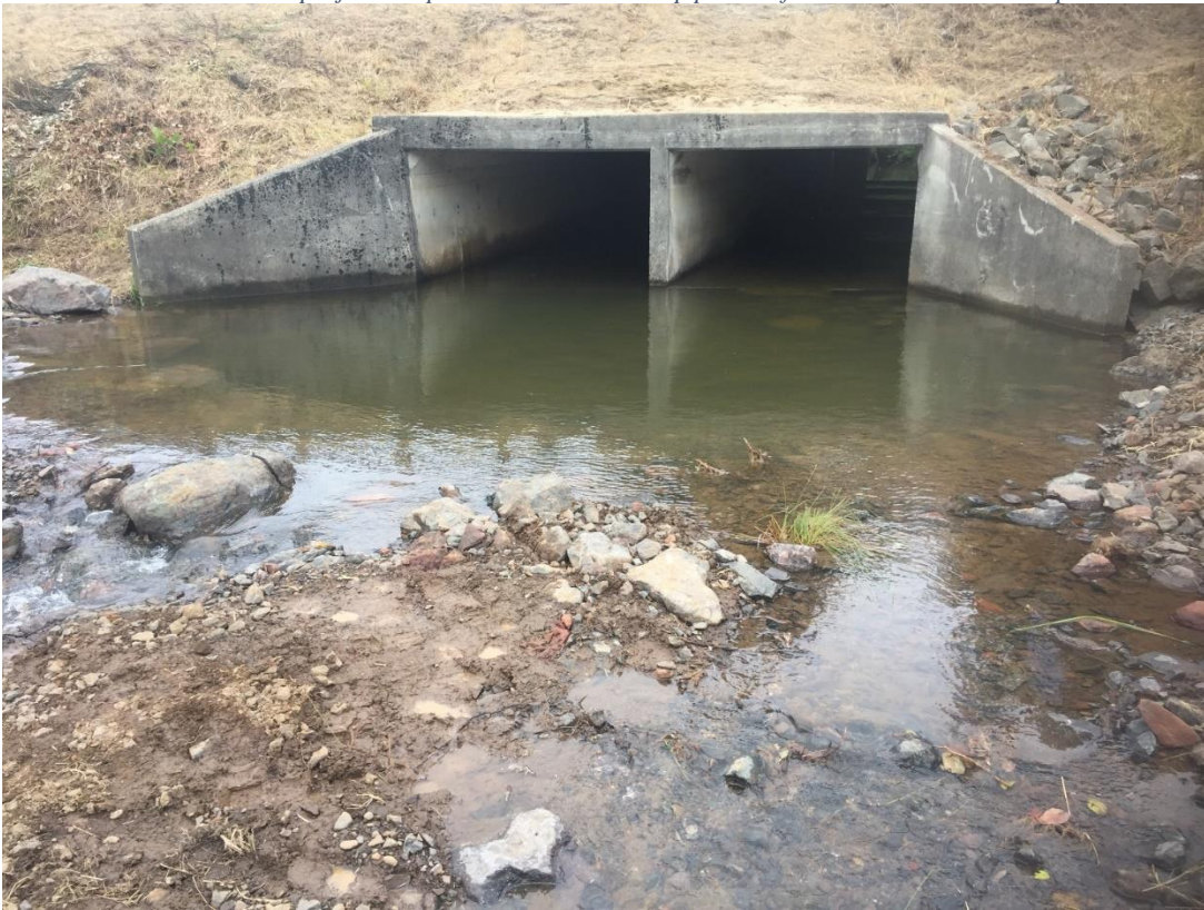
Photo 33- SC#E3 – Modified roughened chute below culvert jump pool. 10-11-2017
