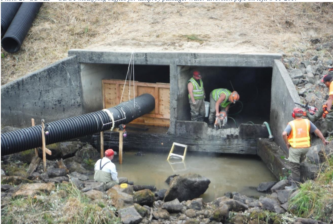
Photo 29- SC #E3 – ODOT modifying baffles for lamprey passage. Water diversion pipe on left. 8-11-2017
