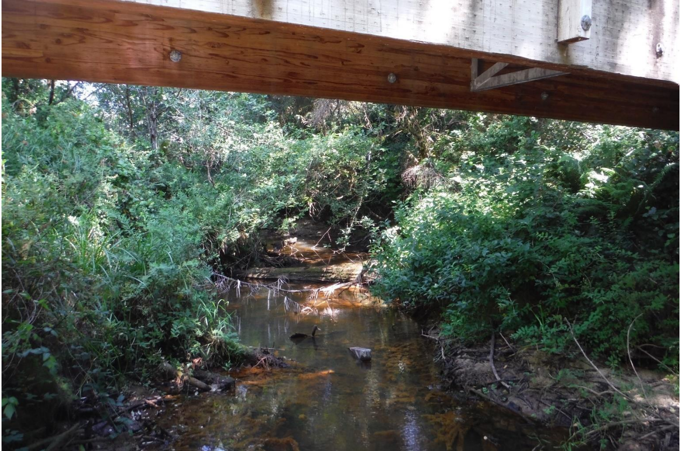
Photo 41- SC#E8 – Foot bridge in Tugman State Park
