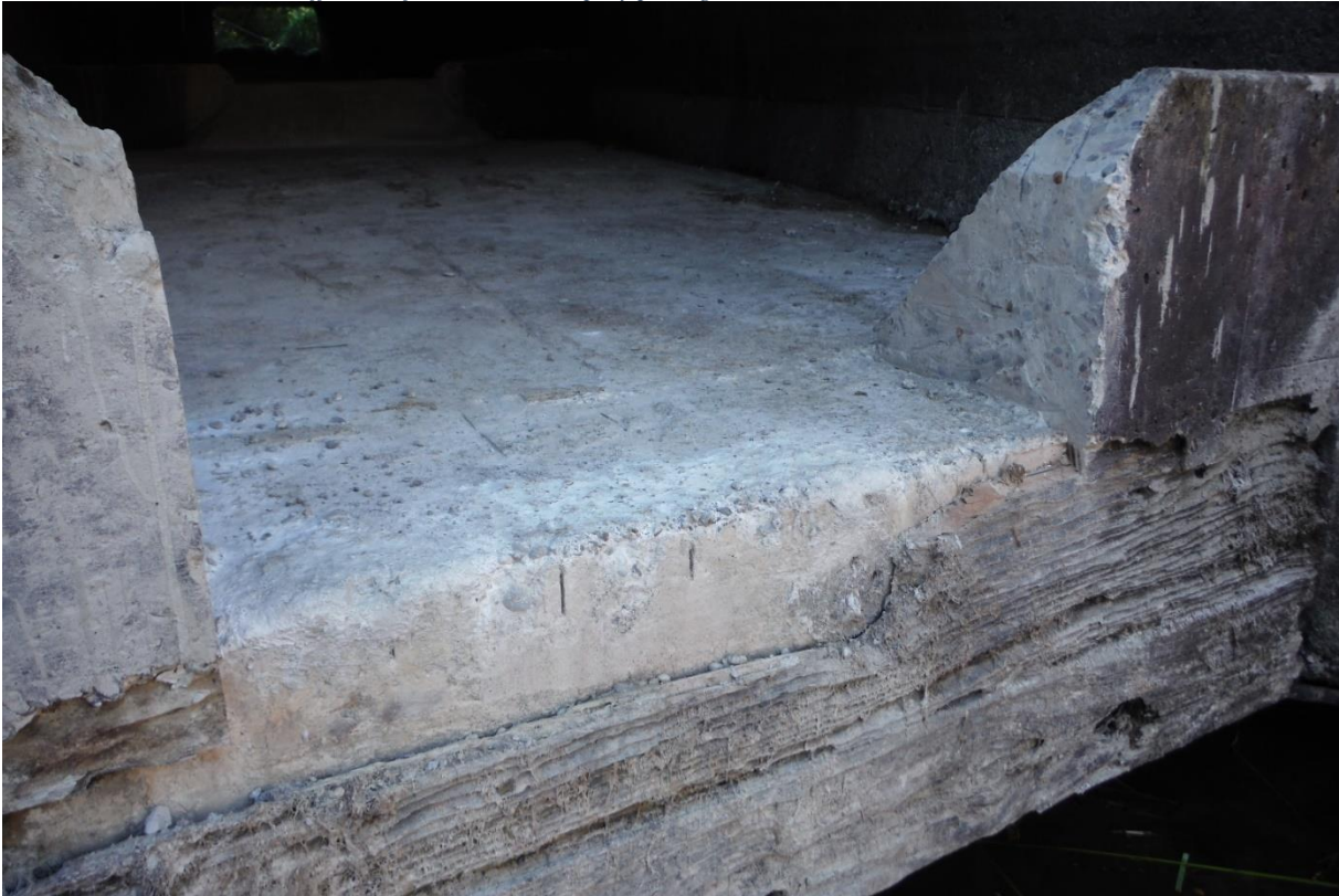
Photo 31- SC#E3 – Concrete ramps poured for lamprey passage on interior baffles. 8-15-2017
