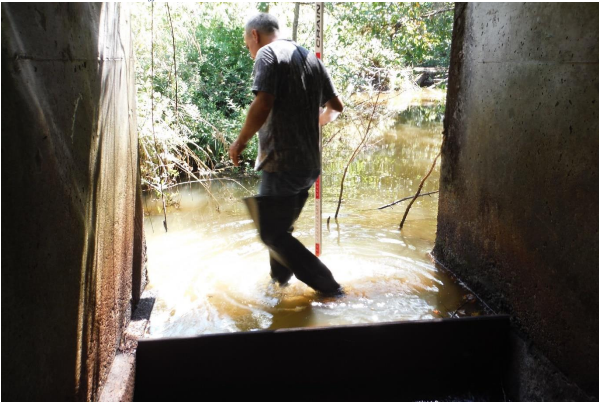
Photo 37- SC#E6 – Interior baffle
