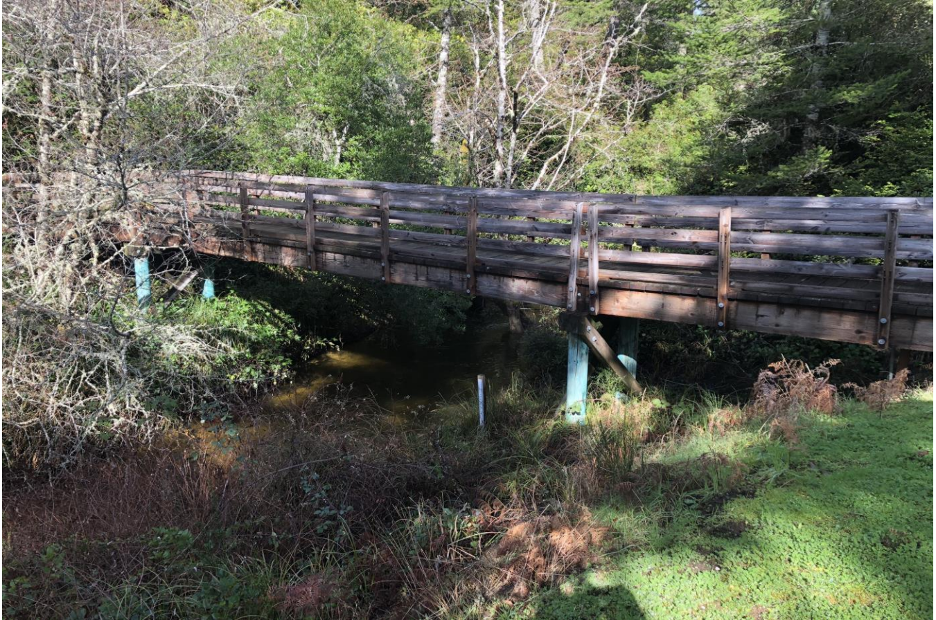
Photo 34- SC #E4 – Walking Bridge
