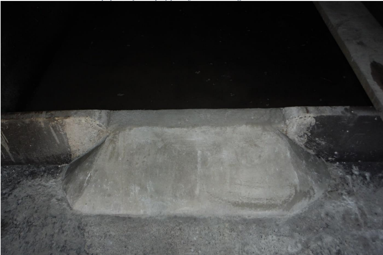
Photo 31- SC#E3 – Concrete ramps poured for lamprey passage on interior baffles. 8-15-2017
