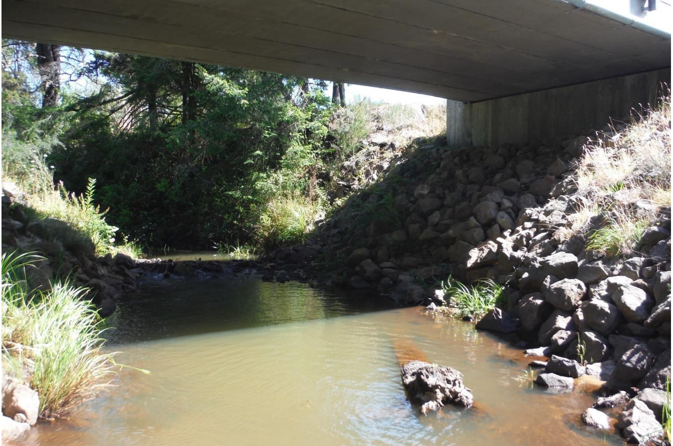
Photo 35- SC #E5 – Bridge at Eel Creek Campground Entrance
