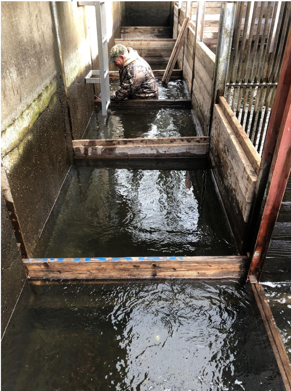
Photo 58- Eel Lake Trap Conversion to Fish Ladder
